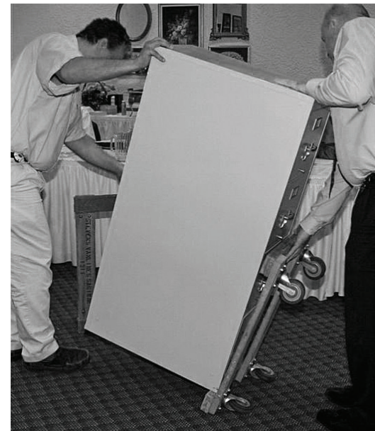
The “shotgun” method for placing cabinets onto dollies
